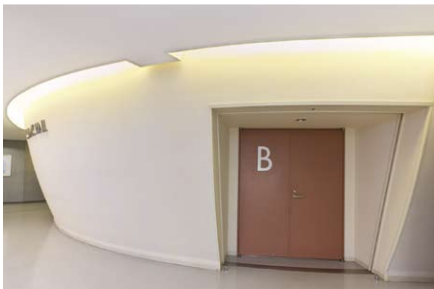
Osaka Mode Gakuen/HAL Osaka FG Board on spherical exterior of Main Hall
