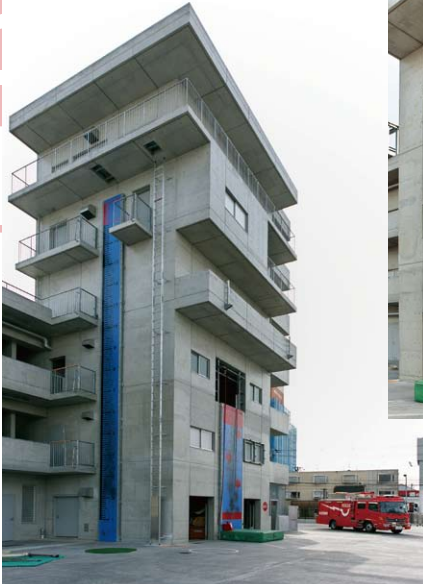
Higashiosaka City Fire Department Training wall Guard Panel N Used for abseiling practice and other training activities
