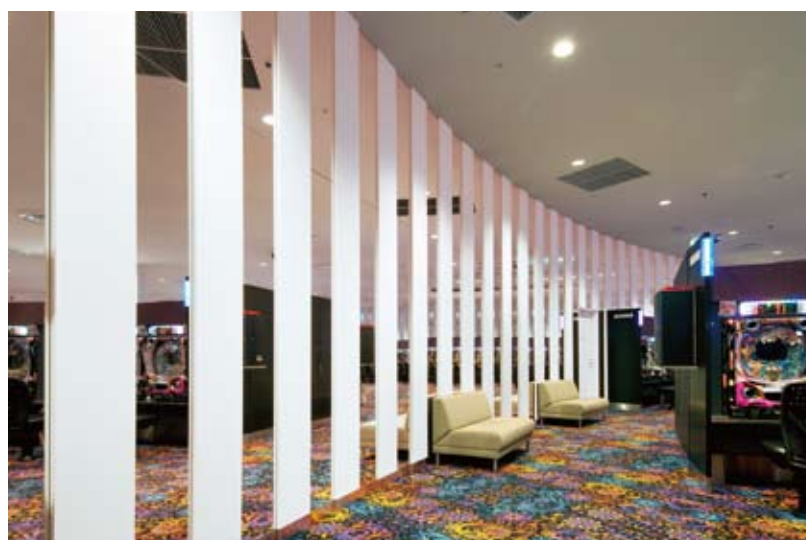
Maruhan Kamiotai Station Branch Interior walls FP FG Board (decorative finish, partially covered with mirrors)
