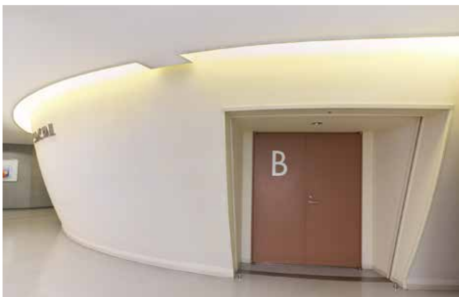
Osaka Mode Gakuen (HAL Osaka General Campus) Interior walls of external section of sphere FG Board
